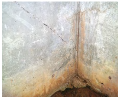
Cracks in perimeter beams
