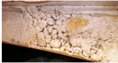
Honeycombing around access hatch
