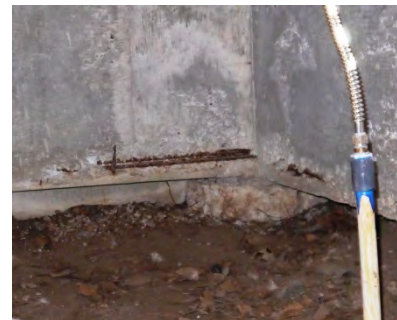
Exposed rebar at bottom of perimeter beam
