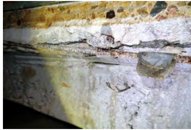
Exposed rebar around access hatch
