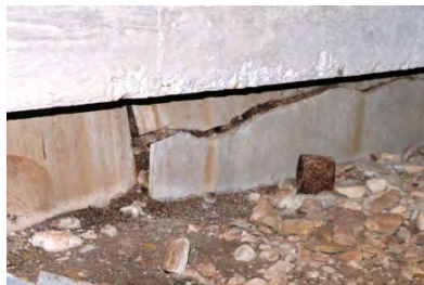
Cracked soil retainers
