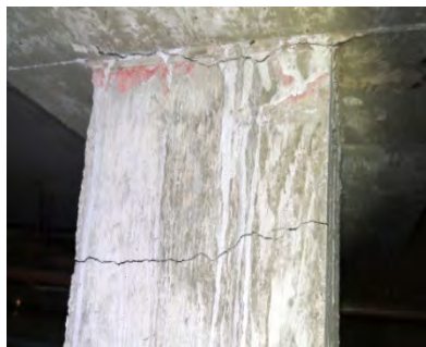
Crack on inside face of column
