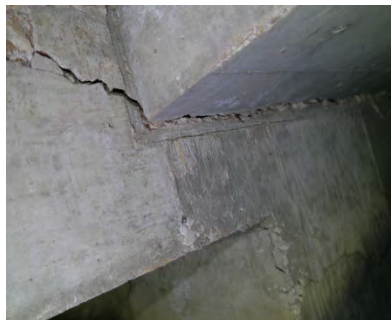
Cracking at exterior and interior beam connection
