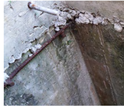
Exposed rebar around areaway
