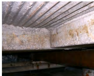
Honeycombing on interior beams
