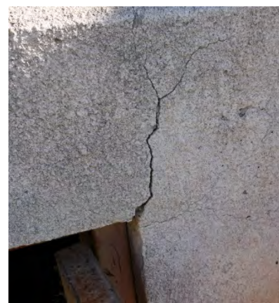
Cracking at corner of access hatch
